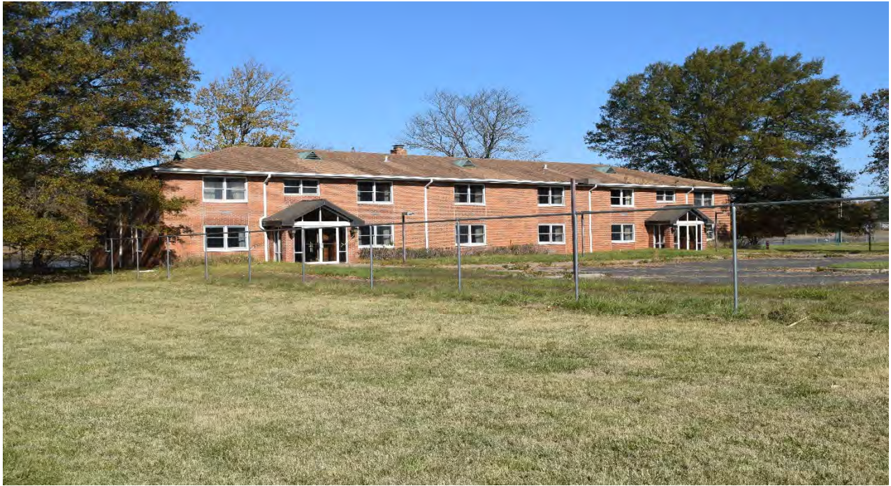
Photograph 5: Northern view of building 364, with Parkers Creek in background
