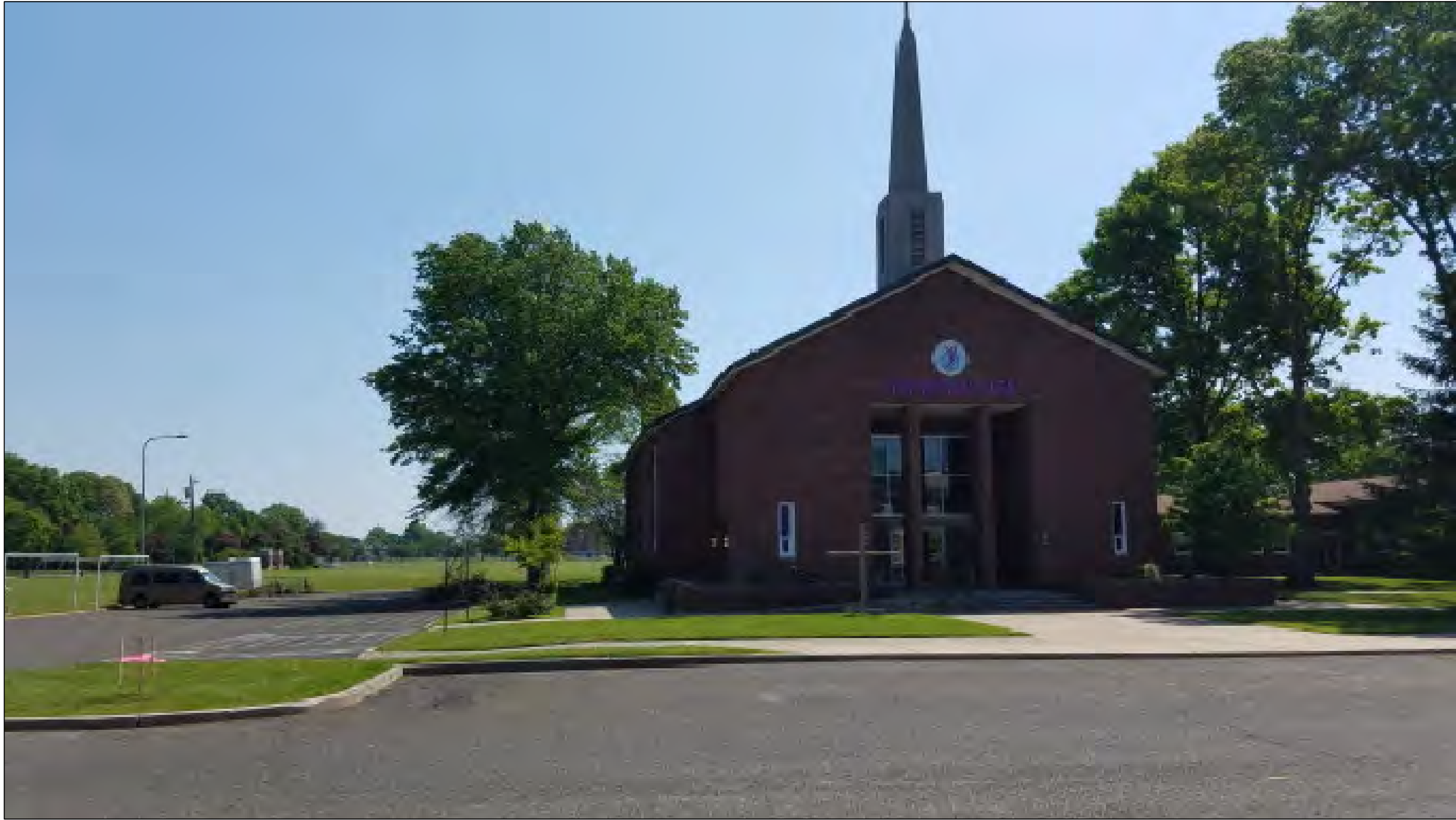
EXISTING FRONT VIEW
