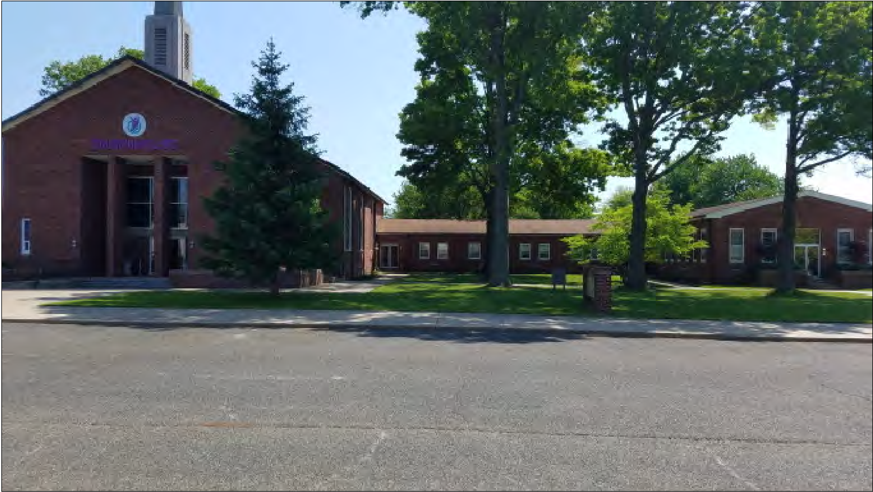
EXISTING FRONT VIEW
