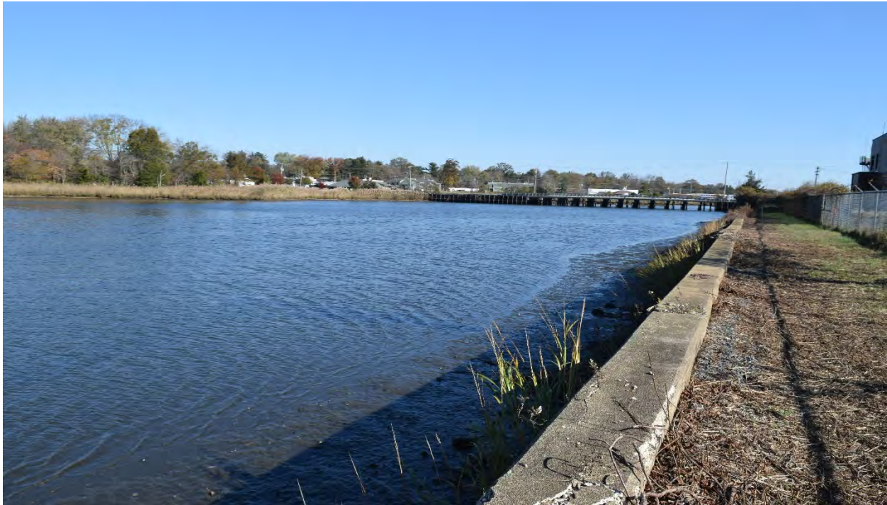
Photograph 1: Northeastern view of Parkers Creek, bulkhead, and a coastal wetland fringe adjacent to the bulkhead.
