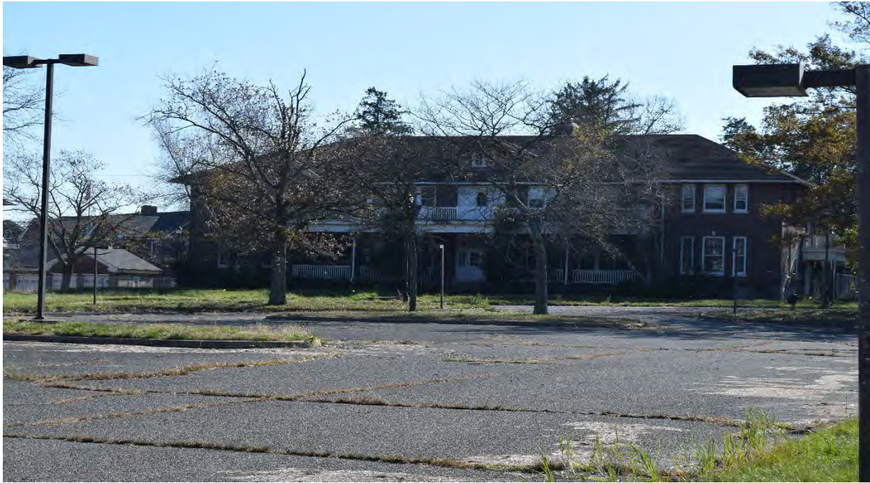
Photograph 7: Southern view of the parking area for building 363 (foreground) and Signal Avenue and building 271
