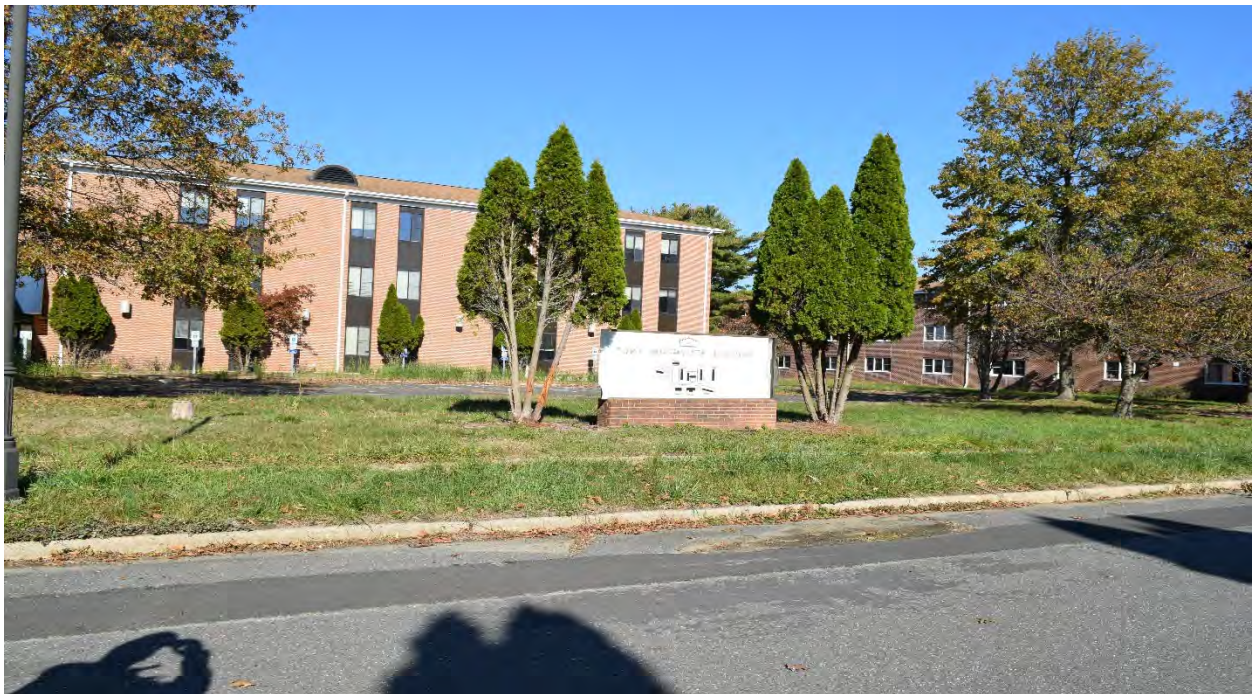
Photograph 8: Northern view of Signal Avenue and buildings 365 and 362
