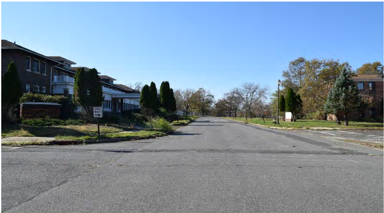
Photograph 6: Southwestern view of Signal Avenue and buildings 270 and 271 on left side of road, building 365 on right
